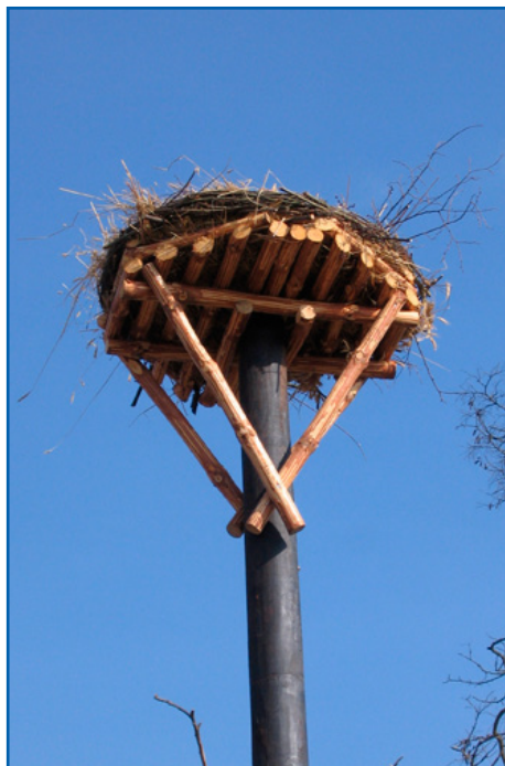
The method of mounting a universal nesting platform on a wooden pole. Photo: AT
