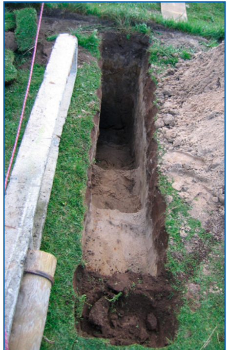
Stepped trench making it easier to set up a pole. Photo: AT
