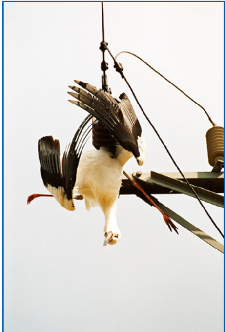
An inadequately secured pole can be the cause of death of many storks. Photo: MR
