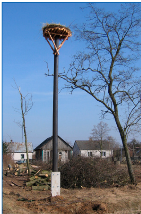
Wooden pole on a concrete stilt with a platform. Photo: AT
